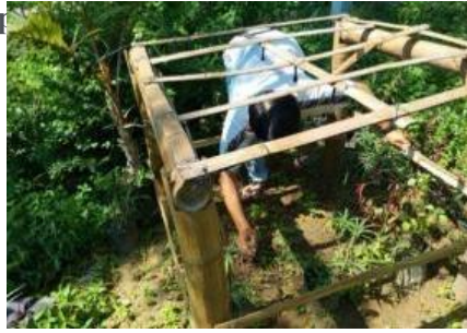
Figure 3. Equipment installation activities at the “Kamila Garden” flower stand
