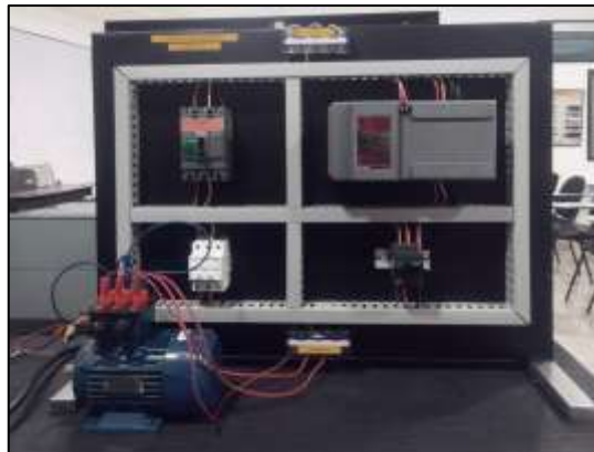
Figure 3. Physical realization of the three-phase electric motor monitoring and protection prototype
